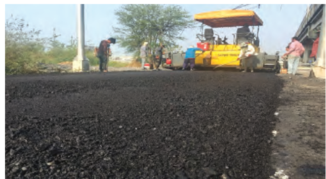
The plastic road phase 2 at the connecting exit road to the motorway with 250 meters length and 6 meters wide or 1,500 square meters.
