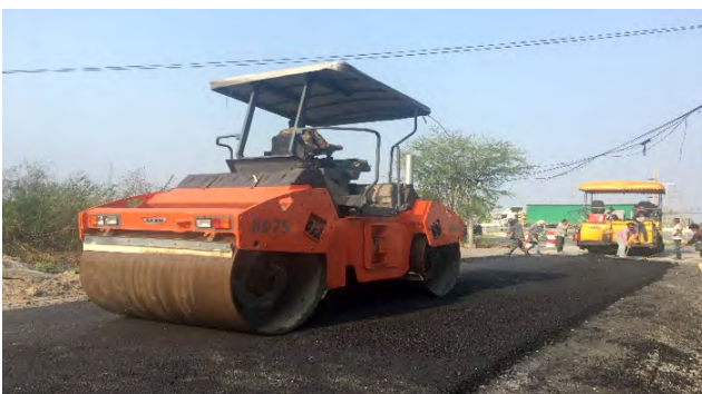
The plastic road phase 2 at the connecting exit road to the motorway with 250 meters length and 6 meters wide or 1,500 square meters.
