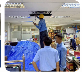
Replace existing air-conditioning units with high-efficiency models (Energy Label No. 5 / high SEER) at the AMATA Service Center building, Chonburi office
